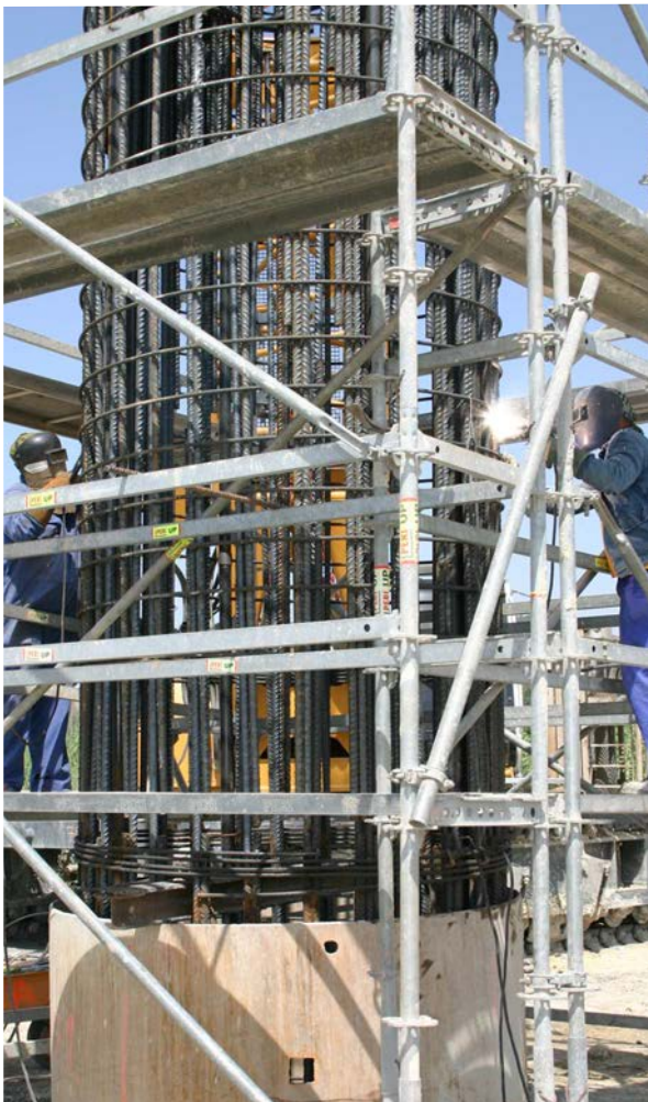
Overlapping and fitting of pile reinforcement
