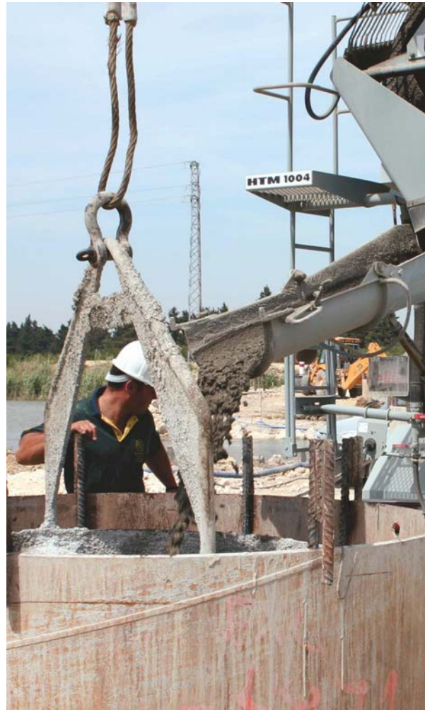
Concreting piles using tremie tube
