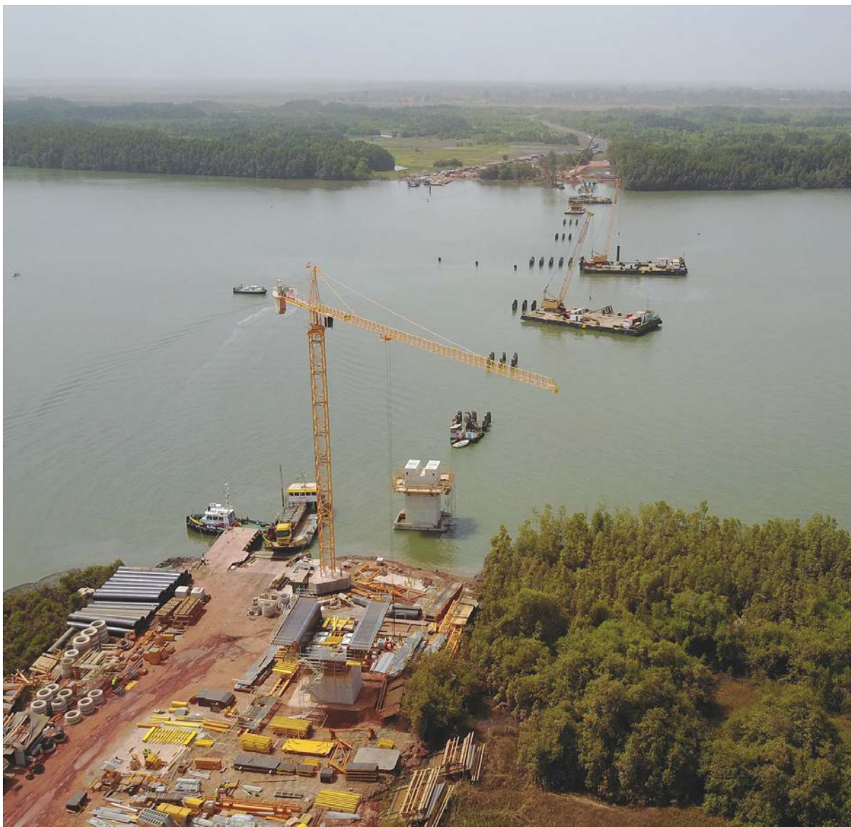
Steel Piles Trans Gambia Bridge (The Gambia)
