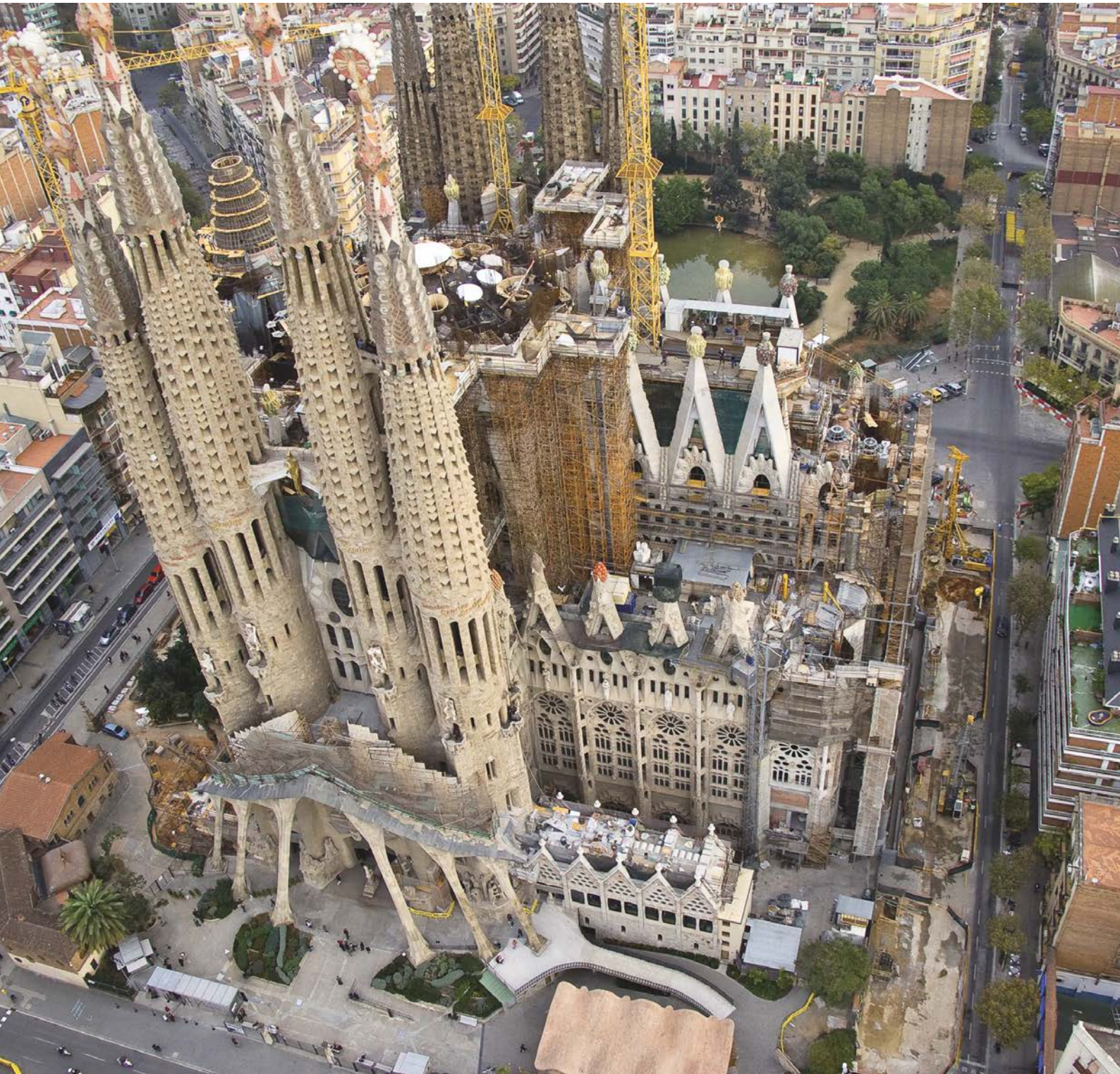
Madrid-Barcelona-France Border High Speed Railway, Spain
