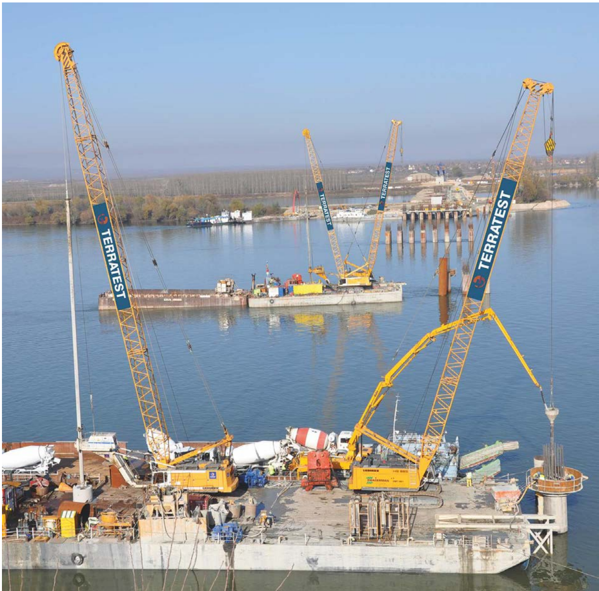
Danube River Bridge Vidin (Bulgaria) Calafat (Romania)
